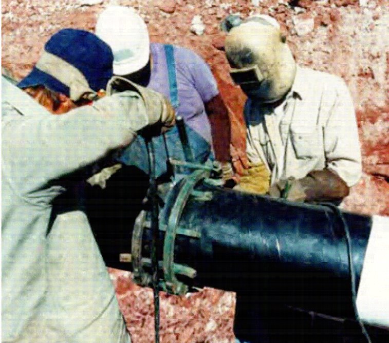
Rapid alignment can be achieved with the Hand Lever Cage Clamp. A Clamp is needed for each pipe size to be aligned.
