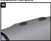
The CFS has been fully installed when adhesive can be seen around the entire circumference. Visually inspect that the patch for any breaks or holes.
