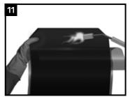
Partially remove the release liner [approximately 1 metre (3') from the edge] from the corner trimmed sleeve edge.
