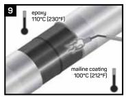
Preheat the epoxy to a temperature of 110°C (230°F) and the abraded mainline coating to be covered by the sleeve to a minimum of 100°C (212°F) with the appropriate propane torch, induction heating or infrared heating equipment. **Do not use an intense flame on the mainline coating.** If a film develops on the mainline coating because of preheat, use a surface abrasion tool to remove it.
