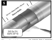
Warm the joint area to 40-50°C (104-120°F) before grit blasting. During high winds or cold ambient conditions (below 15°C (59°F)) prewarm the joint area to 70°C (158°F) before grit blasting. Thoroughly clean the weld area with a sand or grit blaster to "near white metal" SIS Sa 2½ or equivalent. Abrade the mainline coating adjacent to the weld area to a distance 50mm (2°) beyond the sleeve width.
