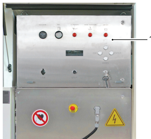
Figure 7.3 - Check the correct execution of the automatic test in the generator power supply phase
