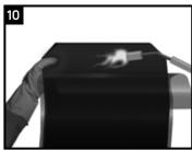
Partially remove the release liner and gently heat the underlap approximately 150mm (6") from the edge. Sleeve temperature shall be at least 18°C (65°F) at time of installation.
