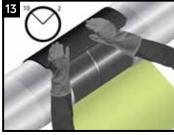
Place the underlap of the sleeve onto the joint, centering the sleeve such that the sleeve overlap is positioned at either the 10 or 2 o'clock position. Press the underlap firmly into place. For J-Lay installation, use Canusa sleeve stabilization bracket to maintain sleeve in the vertical position. Optional spacers can be inserted under the edge of the sleeve to minimize the potential of air entrapment.
