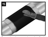
Press the closure and overlap firmly into place. It is strongly recommended that protective heat shields are wrapped around the pipe beside the ends of the sleeve to prevent waxing of the mainline coating.
