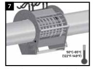
Using the appropriate sized induction coil or propane torch, pre-warm the steel area to 50-65°C. Using a temperature measuring device, ensure that the correct temperature is reached on the steel.
