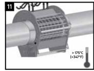
Carefully, move the induction coil into place and pre-heat the epoxy coated cutback to a minimum of 175°C. Preheat temperature and profile is dependent on project specific conditions, and must be determined prior to the start of project.
